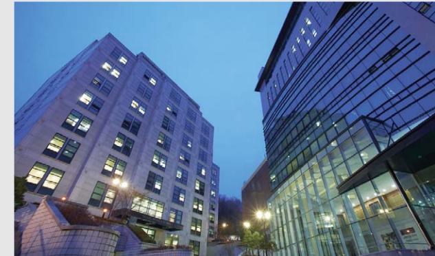
(SBS Main Building)
